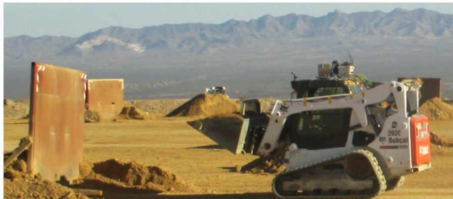
Bobcat T650 with EDAQ processor connected to roof and many sensors attached.
